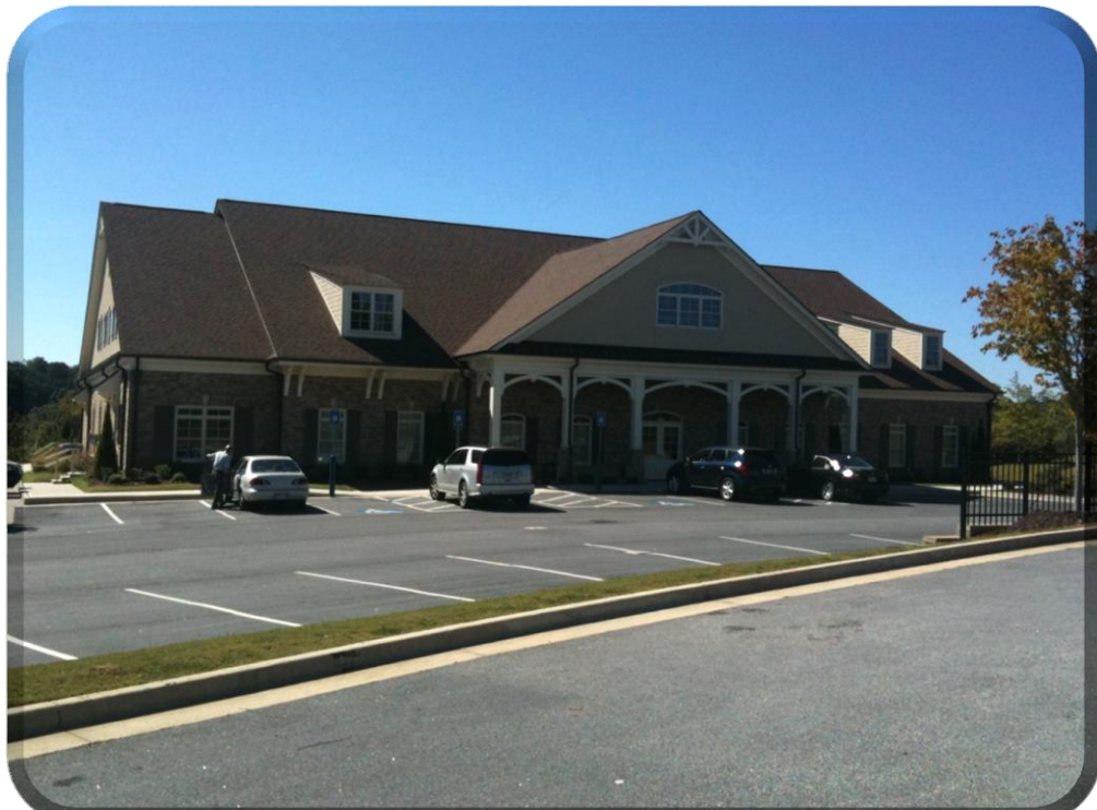
The brand-new building that houses the Lanier Interventional Pain Center sits on Lots 8 and 9.
