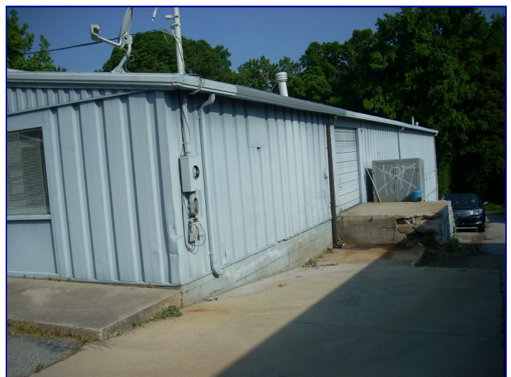
Side loading dock serving main floor.
