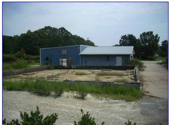
Side view of 2,100 s.f. building.
